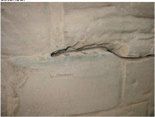
Consolidation by Grouting - Here a degree of ingenuity has to be performed. The wall may be voided as in many cases with a random stone cored wall. The wall is checked for integrity with optical probes and a decision made whether the core is capable of receiving grout.
