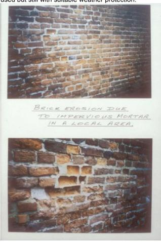
It should always be remembered that 'hard onto soft' will not work. Often one sees 'new' shallow pointing falling off the front of the joints. This is not only because it was shallow but in application the joint may not have been 'wetted in or cured' properly. Any mortar if cementitious or stronger it has a greater potential for shrinkage and is loosened on initial drying out. Pinch points can be caused with a hard mortar putting stress on the hard fired brick edges.
